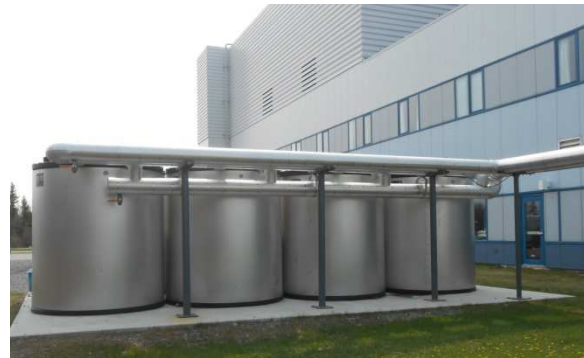
Chiller System Replacement
